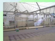
Variable-boarding-location-type Automatic Platform Gate
